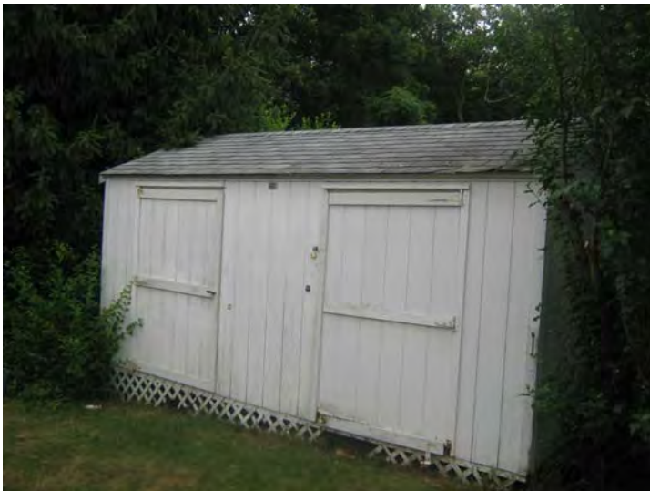
View of typical storage shed – siding noted to be weathered at several locations.
