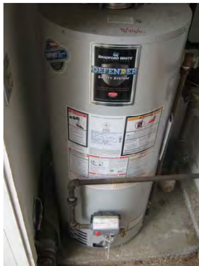
Bradford White natural gas fired domestic hot water heater – 1 hot water heater per unit.
