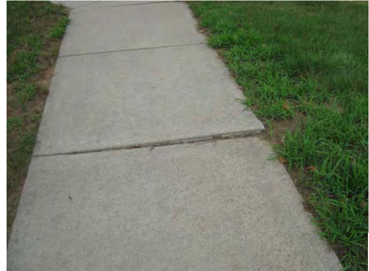
Isolated uneven section of concrete walkway; isolated areas of cracking also evident.
