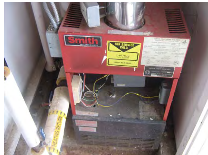
HB Smith boiler for production of hydronic heat – 1 natural gas-fired boiler per unit.
