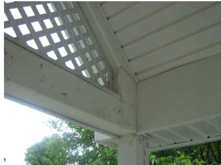
Deteriorated paint finish noted at entrance canopies.
