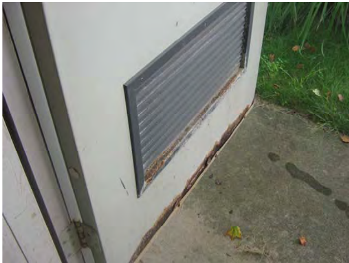
Surface corrosion noted along base of service doorway.
