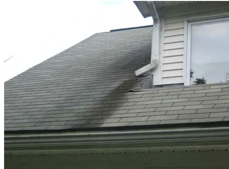
View of staining from water-runoff on composite asphalt shingles.
