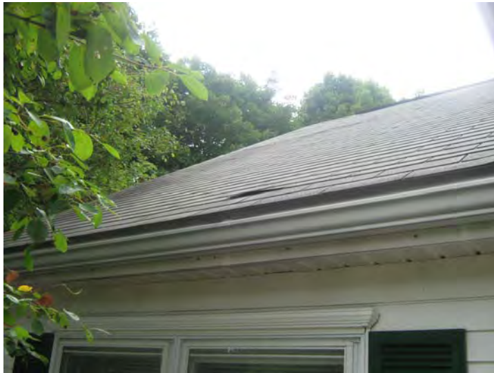
View of poorly adhered composite asphalt shingle.
