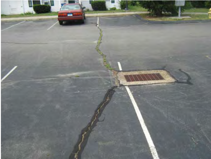
Cracking noted within the asphalt paved surfaces.
