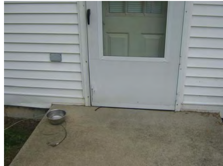
View of damaged rear patio storm door and weather-stripping.
